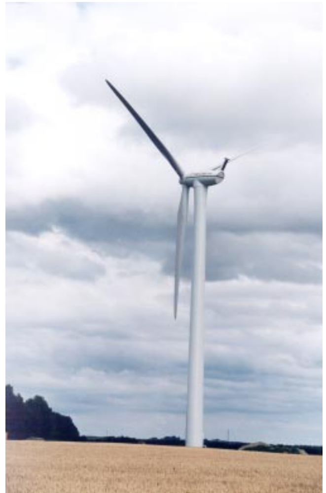
New 2 MW N.E.G. Micon turbine (Photo: Flemming Hagensen)
